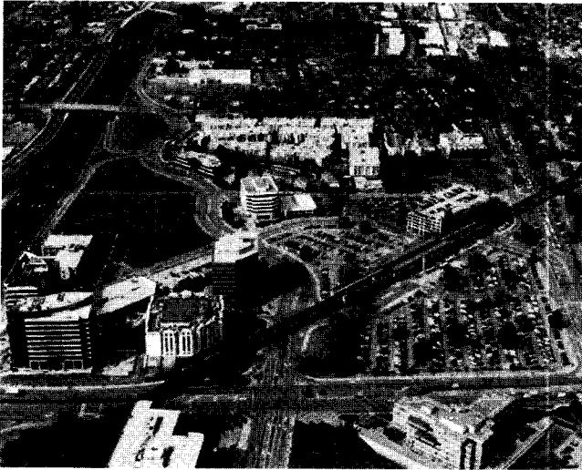
FIGURE 1 Pleasant Hill BART station and surroundings.
